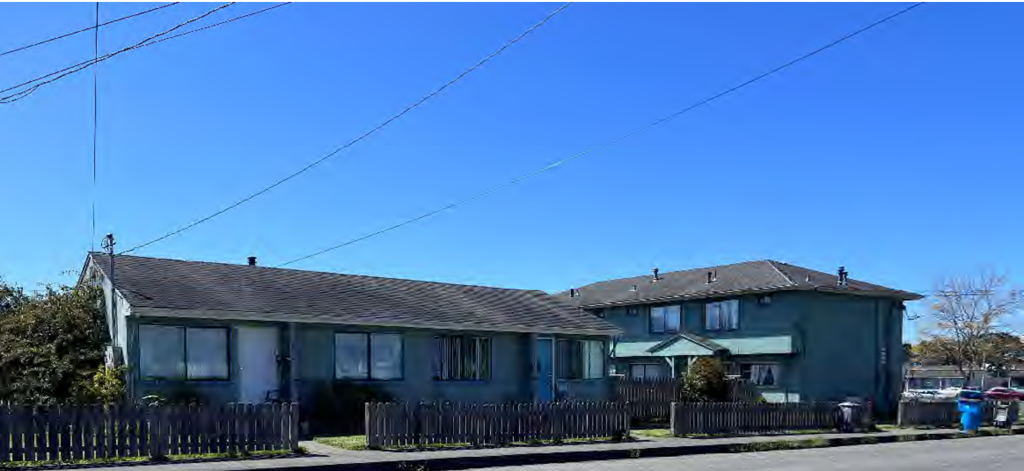
Current Conditions: View from Hiler Street, looking west
