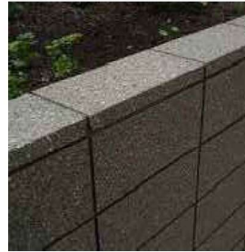
STRAIGHT STACKED CMU RAISED PLANTERS AND PARKING LOT WALLS
