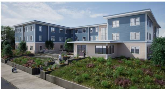
“BLUE & PURPLE PHASE” – 44 UNITS NEW CONSTRUCTION & 4 UNITS REHAB, ALL SENIOR HOUSING
